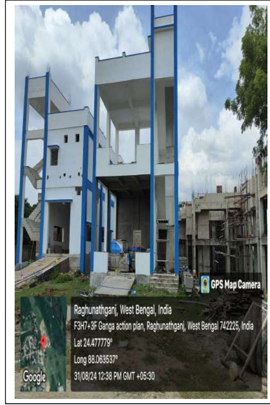
RAGHUNATHGUNJ STP SITE
